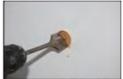
Step 2.... Using the 1-1/8" drill bit, drill a hole through the wall of your pet house (a minimum of 9" from the ceiling) where the center of the Hound Heater will be placed and the power cord will go through.
